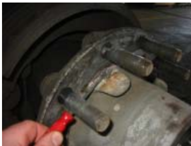
Rust and corrosion build-up.
